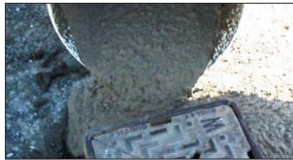
Pouring weber.cem pyracrete
