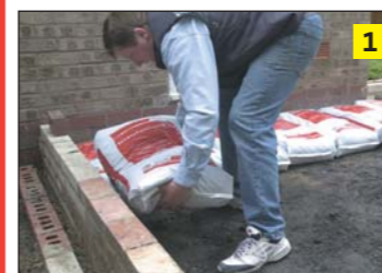
Step 1 Use loose material to level up the sub floor and then lay the bags on top.
